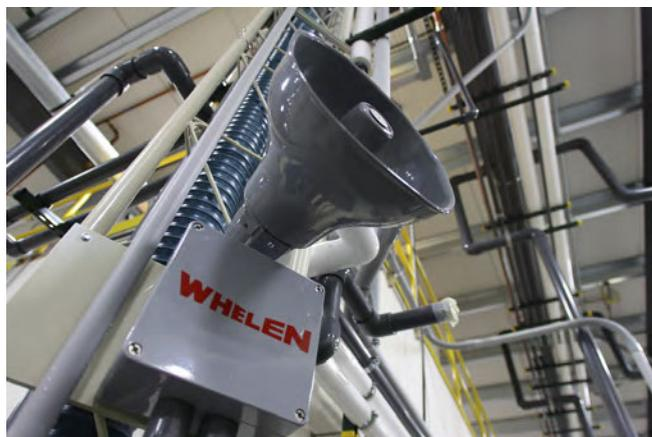
Figure 6: One of seven Whelen-made sirens used to alert employees that a process needs manual attention.
